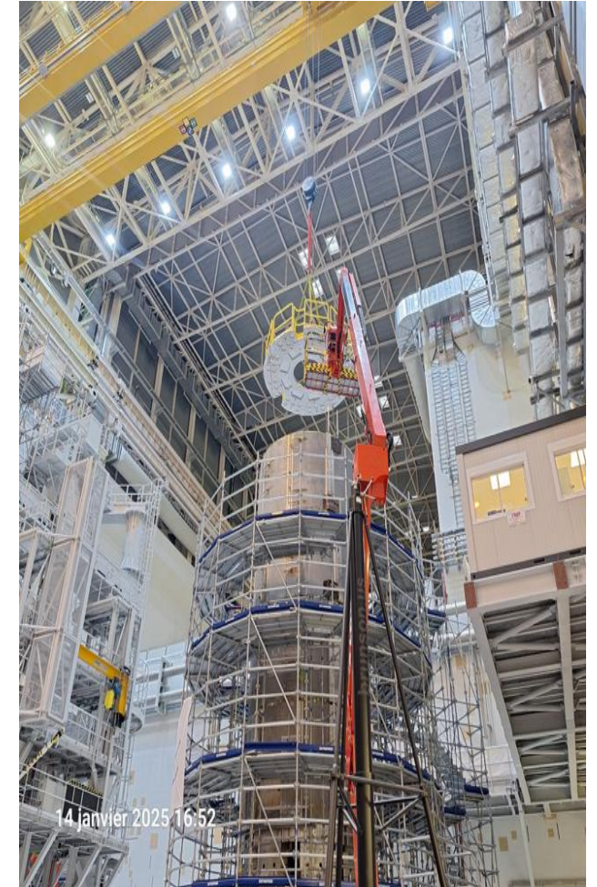
Stacking fourth module, January 2025
