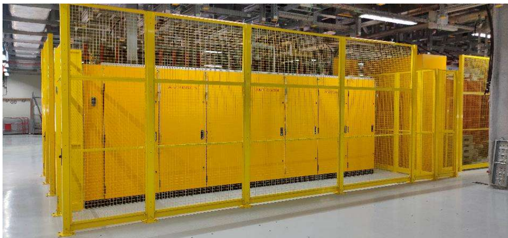
View of the installation of MHVPS manufactured by Ampegon in B15 L2
