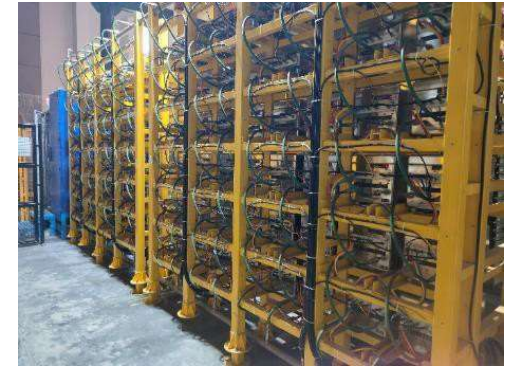
The commissioned 6 MW MHVPS for MW gyrotron cathode circuit at ITER India.
