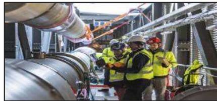
Installation of Seismic decoupling spool
