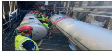
Installation of Seismic decoupling spool
