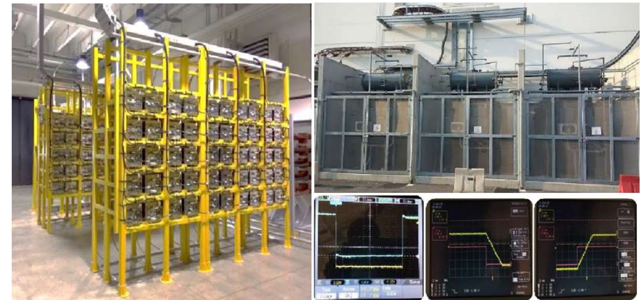
Accelerator power supplies 7.2MW, 100kV HVPS operational at SPIDER facility, RFX, ITALY 100kV Power supply at SPIDER is operational since 2018
