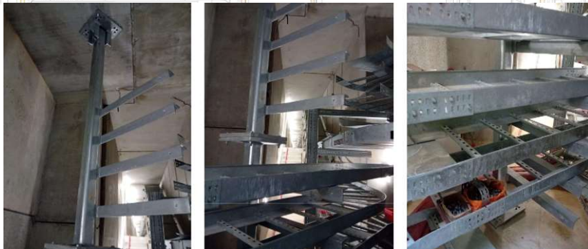
Installation of one of heaviest support vertically
