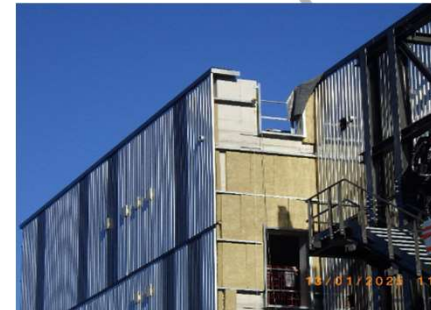
B44 – Cladding installation
