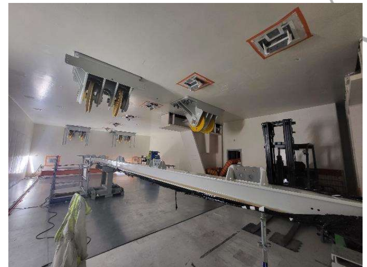
Cargo lift machinery room: 4 upper pulley blocks completely installed
