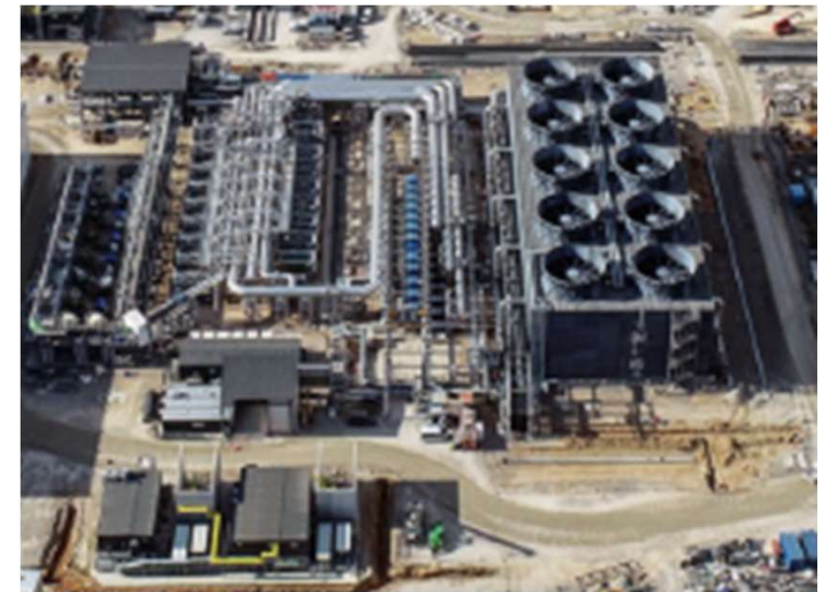
Heat Rejection System & Cooling Water Plant
