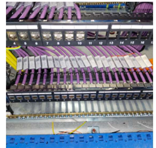
Terminations and Connectors for the Ethernet cables in Main Server Room
