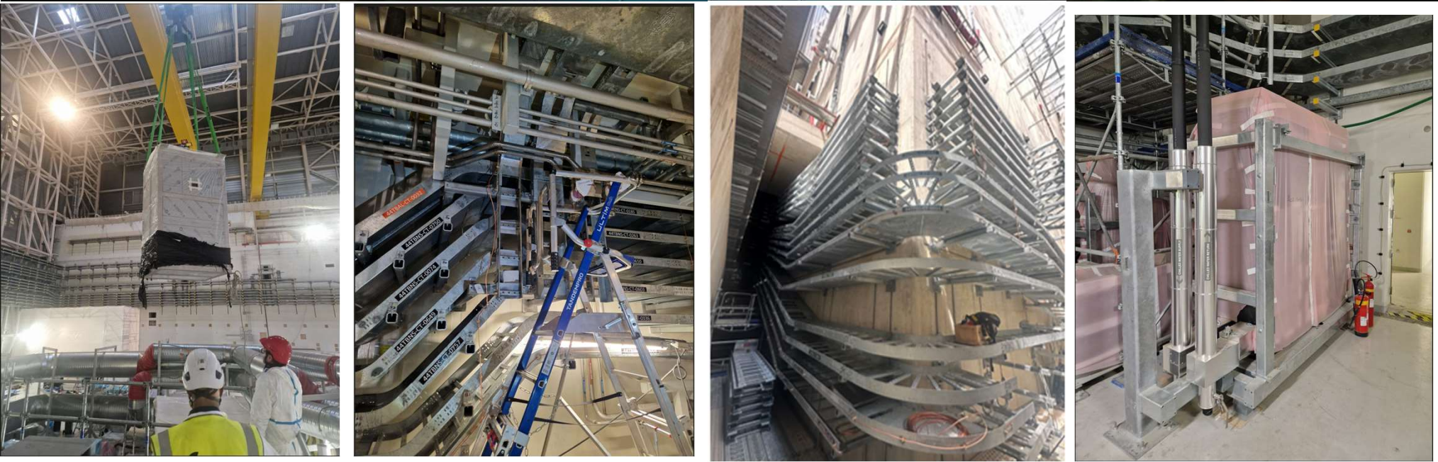
LAC, Cables Trays, HVAC and Piping Installation in B11-B74
