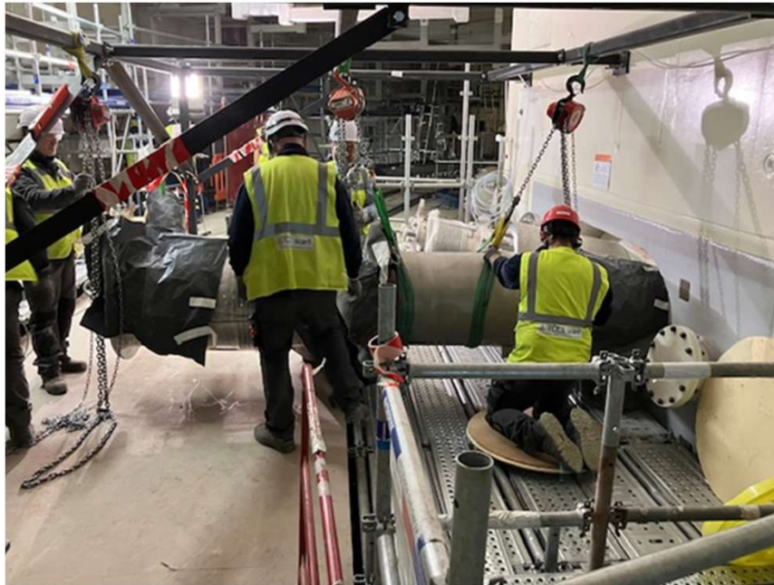
Handling of the TCWS bundles inside a bioshield opening
