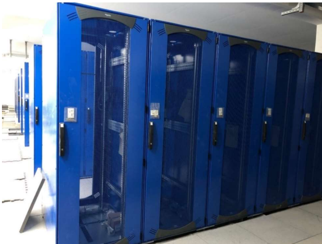
I&C Cubicles in Main Server Room
