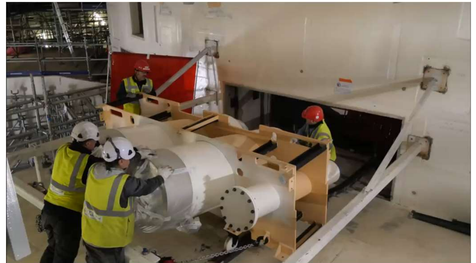
Installation of bioshield openings (structure plus bundles) connecting Work Site 2 to the pit
