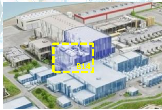
The Tokamak Complex
