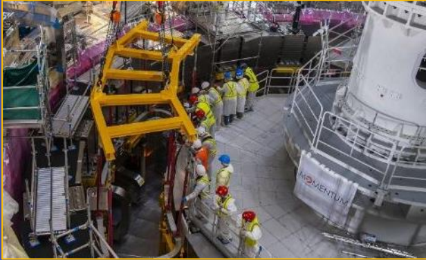
First correction coils installed
