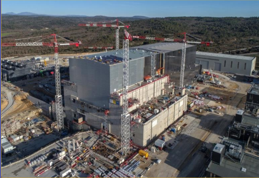
Tokamak Complex, Project Progress March 2020
