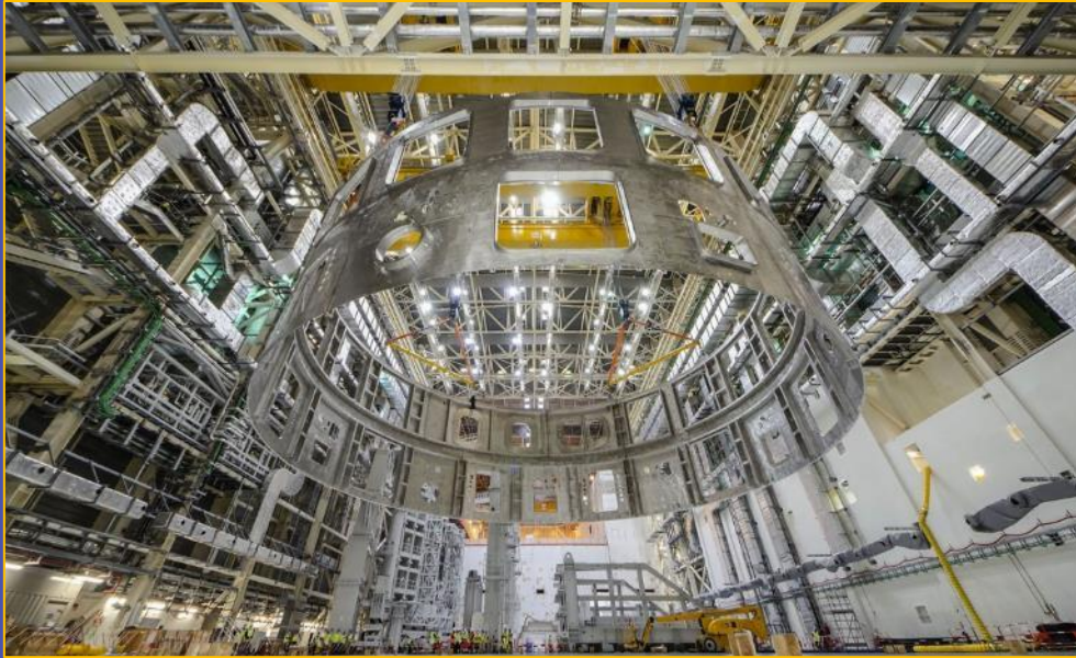
Cryostat Lower Cylinder lift, 31 August 2020
