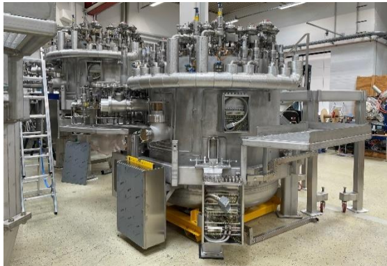
8x Valve boxes: delivery in May 2023
