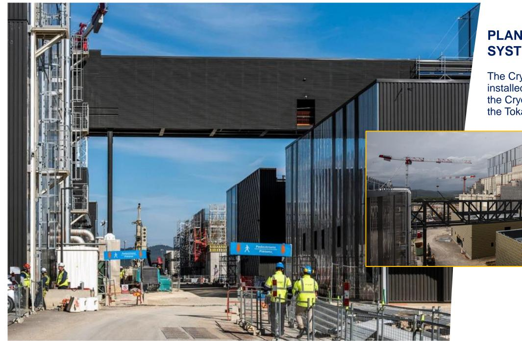
The Cryogenic bridge is installed, now connecting the Cryoplant Building with the Tokamak Complex.
