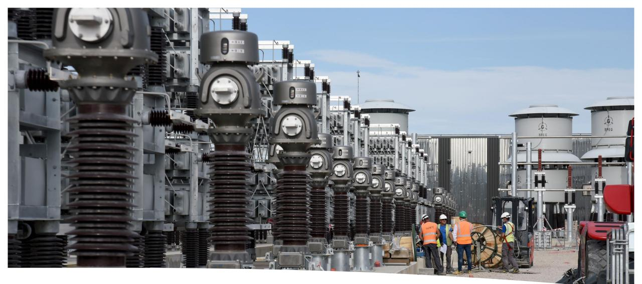
ITER has two overall power supply systems: the steady-state electrical network, commissioned in January 2019; and the pulsed-power electrical system (sometimes called "reactive power compensation"), for which the equipment is largely installed.
